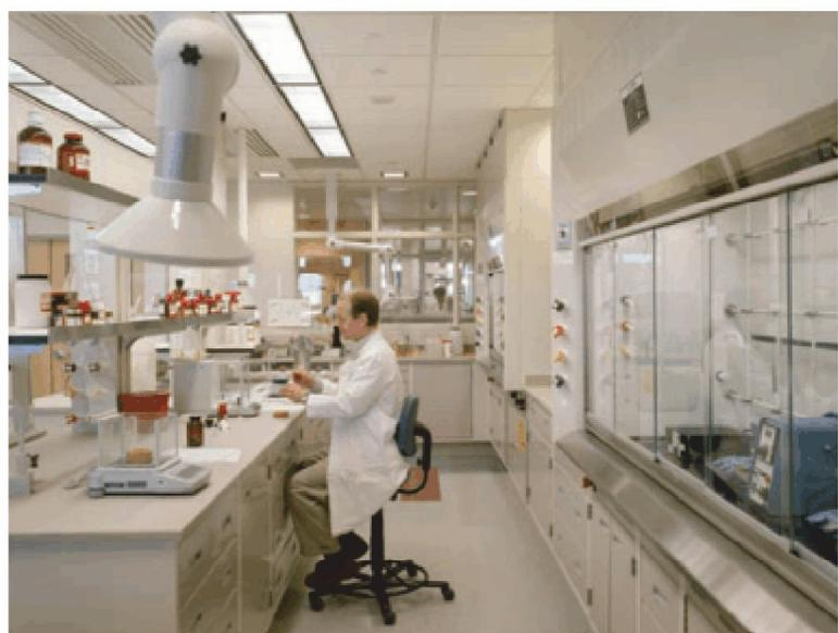
**Figure 10:** Balance of surface brightness in this lab is achieved with energy-efficient recessed lab lighting using T8 technology and compact fluorescent down lights with 4100-K lamp colour.
